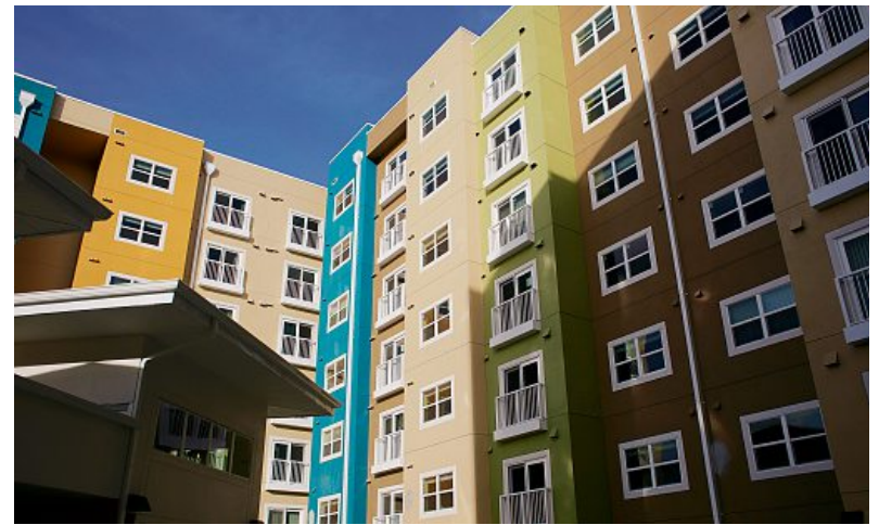
A view of the Ella apartment complex in Tampa, Florida on Thursday, January 3, 2019. After a two-year delay due to legal battles with contractors, one of whom was involved in affordable housing fraud, residents are finally moving into the Tempo at Encore, a public housing building on the edge of downtown Tampa. Times (2019)
